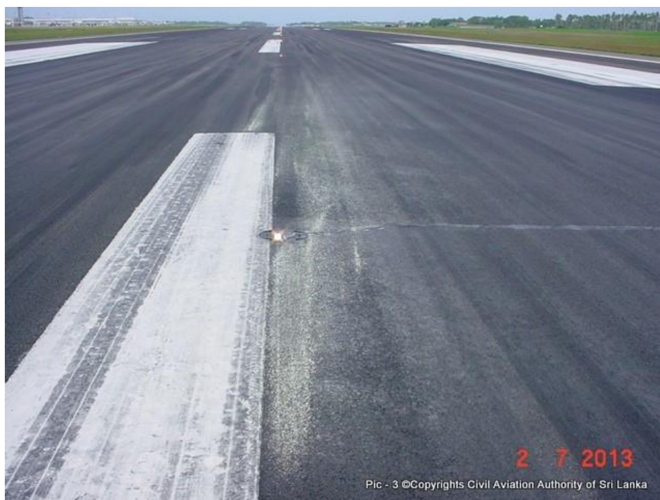
Figure 3 – Runway scratch mark
