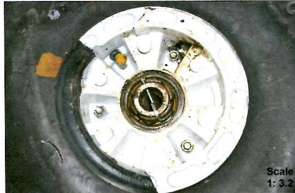
Figure 4: Fractured Rim (View from outside)
