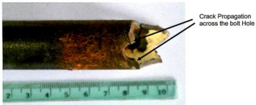
Figure 7: Corroded Remaining part of the Strut with the Crack
