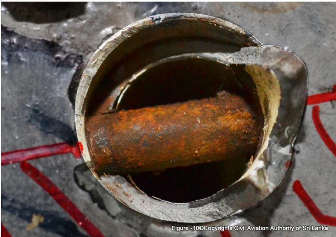
Figure 10: View of damaged Strut
